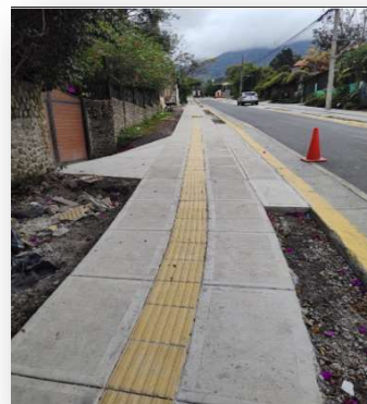
Vereda Peatonal. San Antonio
